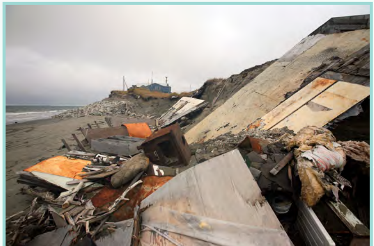
These houses in Shishmaref collapsed because of coastal erosion. Permafrost thaw worsens the problem by destabilizing the shoreline. Photo by GRID-Arendal, www.grida.no/resources/1139
