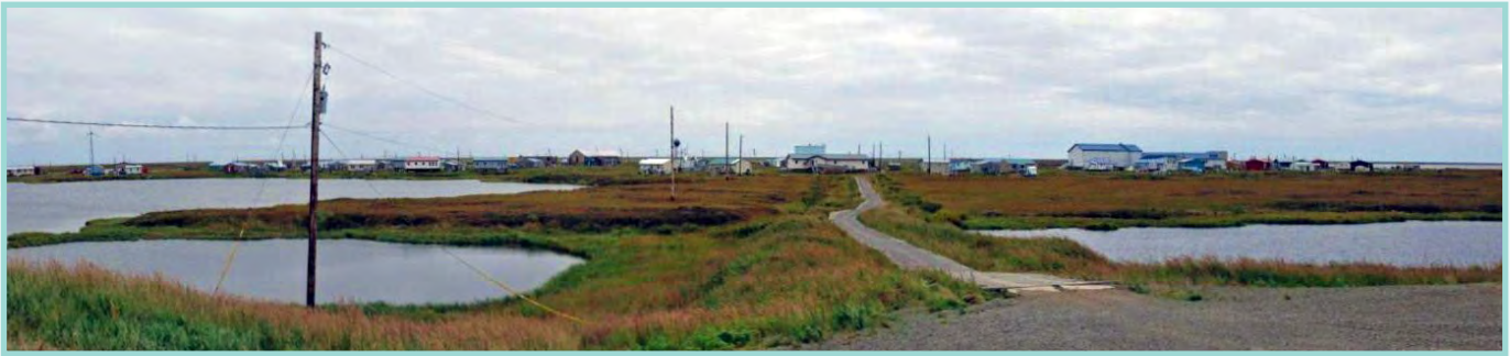
This photo of Newtok was taken in 2010. Boardwalks, such as this one leading into town, are necessary for supporting weight as permafrost thaw makes the ground increasingly soft. Photo by Flickr user Travis
